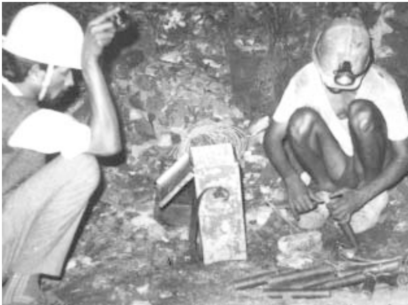
Preparing dynamite sticks for blasting the coal out
